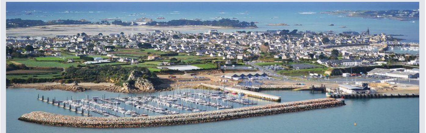
New facilities at Roscoff Harbour, France
