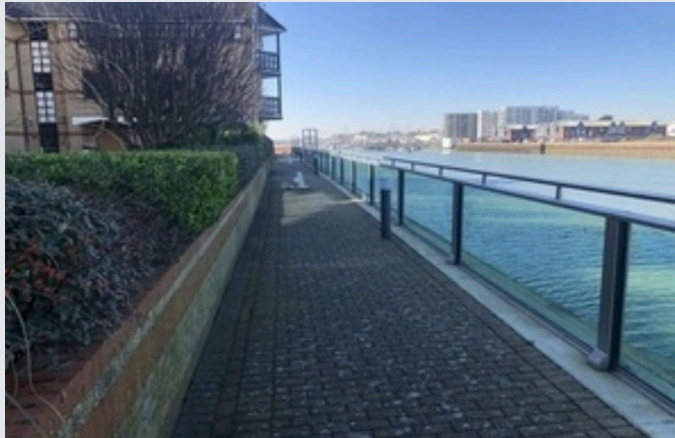
Shoreham glass sea wall (source: gov.uk - https://www.gov.uk/government/news/new-45-million-flood-defence-scheme-for-shoreham-unveiled )
