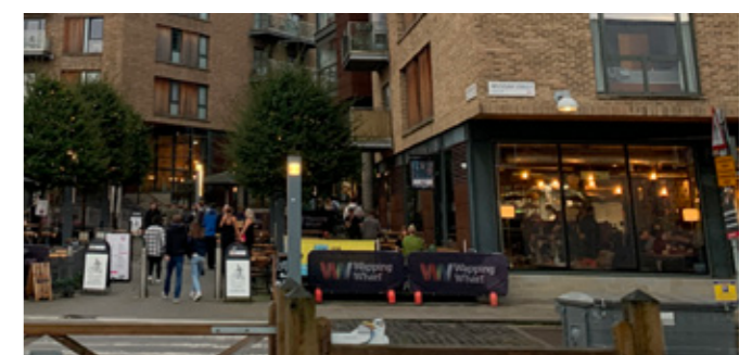
High quality mixed use development at the water's edge, as seen here in Wapping Wharf, Bristol.
