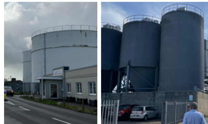
Figure 4.13: Existing fuel storage
