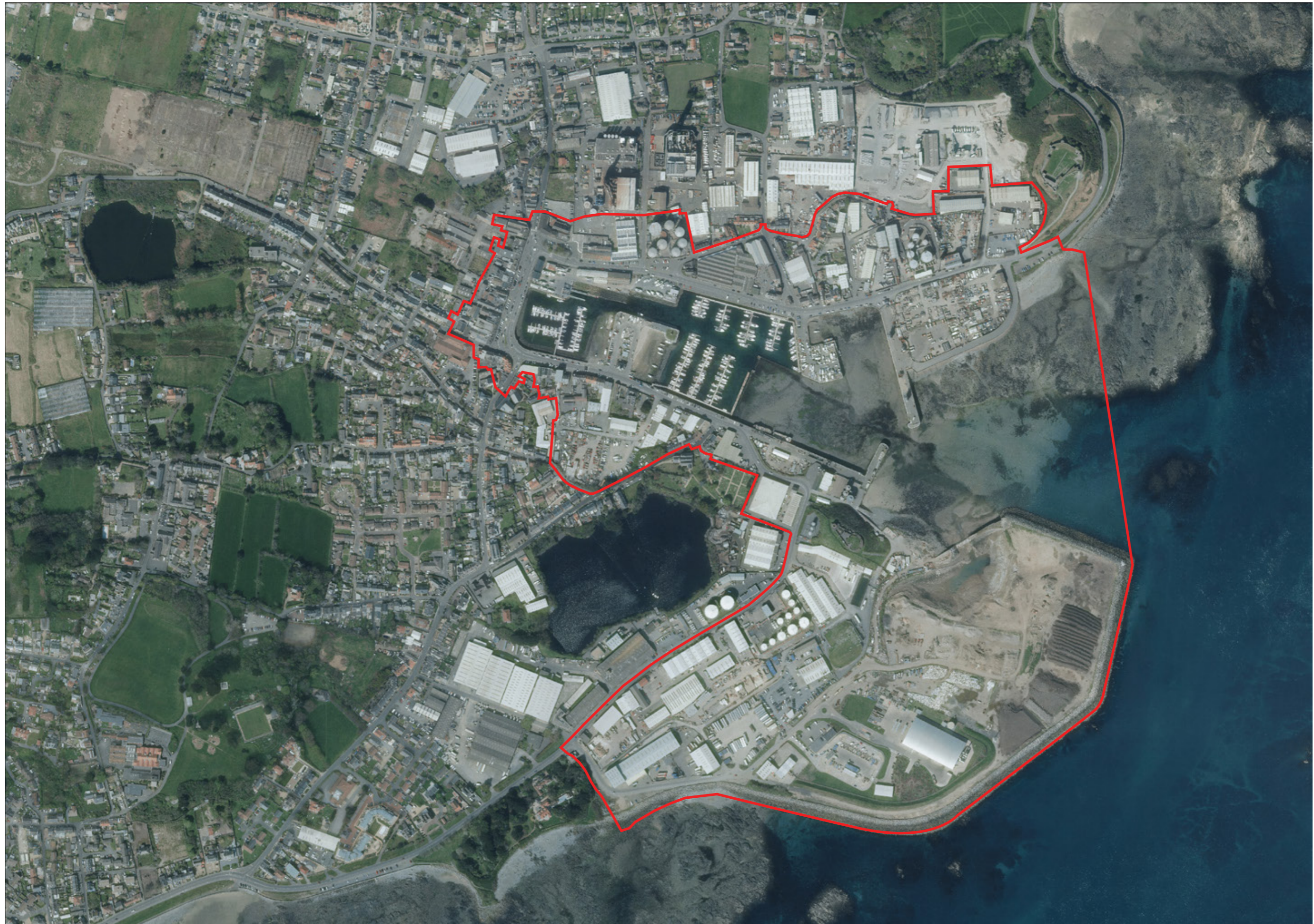
Figure 4.7: St Sampson Harbour 2022
