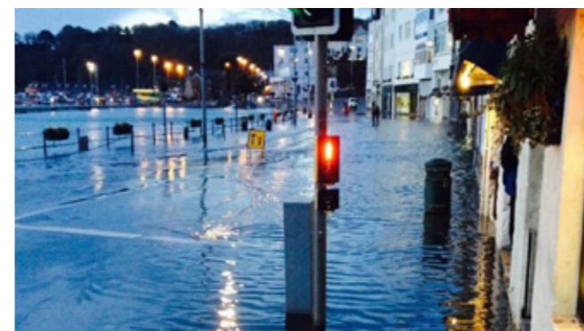
Figure 4.21: Flooding at St Peter Port
