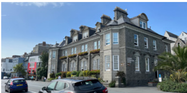
Built heritage is an important asset across the HAAs
